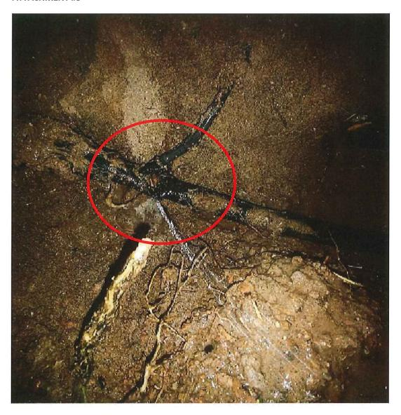
ONE OF THREE SHOVEL CUTS IN IRRIGATION LINE FROM DONA ANA WATER WORK FOR STOP VALVE REPLACEMENT AT METER BOX.
