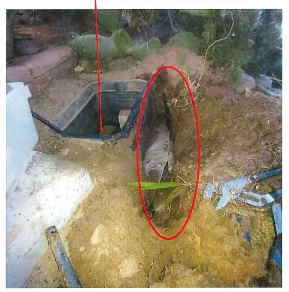
IRRIGATION LINE CUT IN 3 PLACES FROM DONA ANA WATER WORK FOR STOP VALVE REPLACEMENT AT METER BOX.
